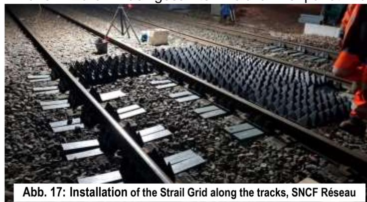
Abb. 17: Installation of the Strail Grid along the tracks, SNCF Réseau
