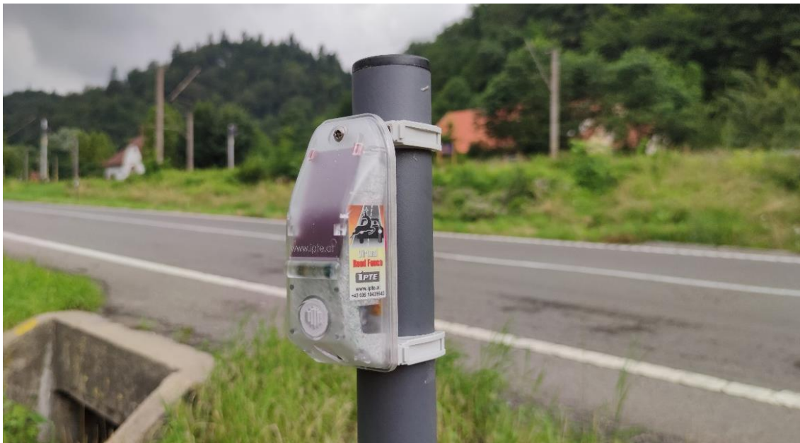
DD430 installation on the E60 south of Braşov (Romania) by the SAFE CROSSING project-team
