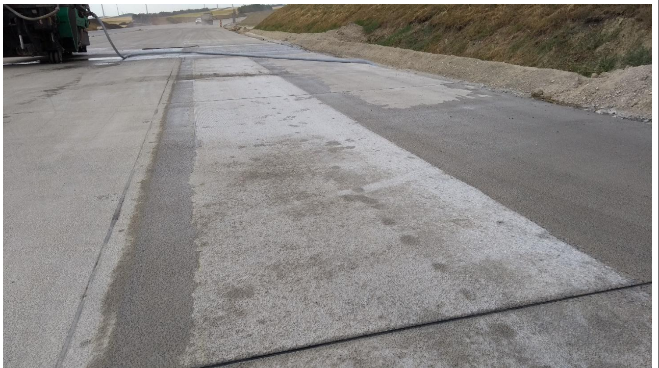
Abb. 2: Grindingfläche 1 Station km 40,625 RF Wien
